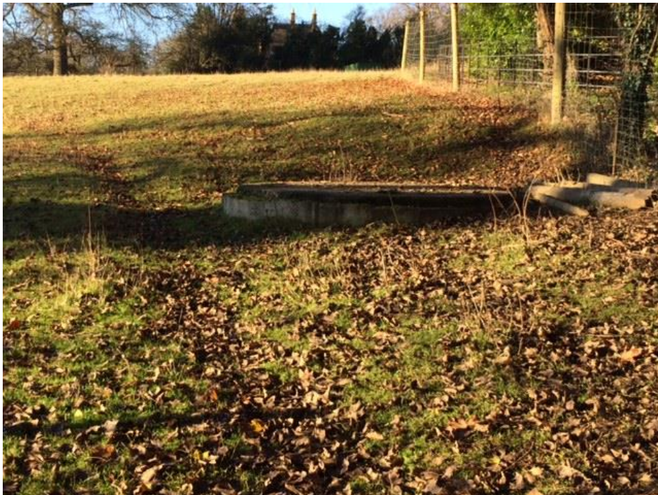
Figure 2: Site of possible sewage system discharge on the west side of the lake
